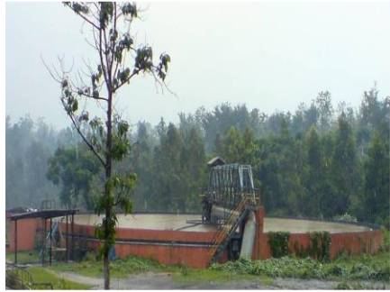
Primary Clarifier - Pulp
